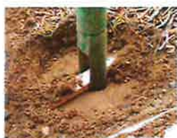
Photo 6: A piece of wood in the auger channel helps clear the soil surface to create a flat base for the Sentricon station. It may also be used to clear lawn, gravel or mulch.
